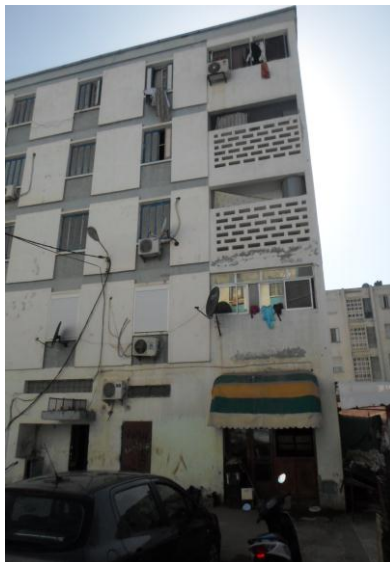
Figure 3: Example of ‘closed’ balconies
