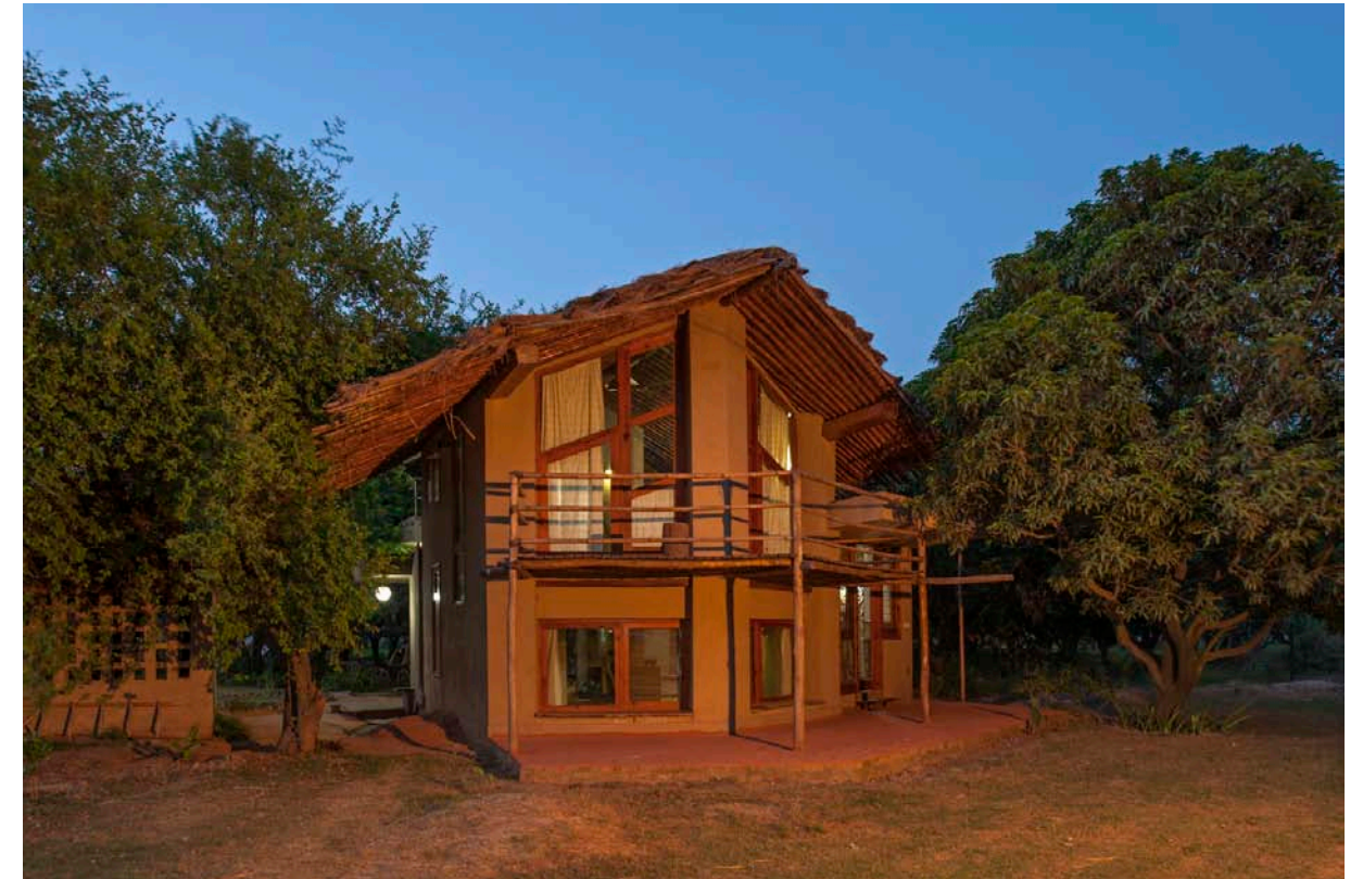
Figure 5 → View from the South West
