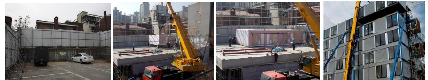
Figure 6. Modular Field Construction Case
