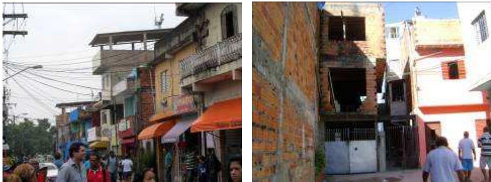
Figures 9 and 10 On the left, view of a typical street within the fabric of Favela Morro da USP . On the right, view of multistorey buildings supported by concrete columns and beams with brick walls.
