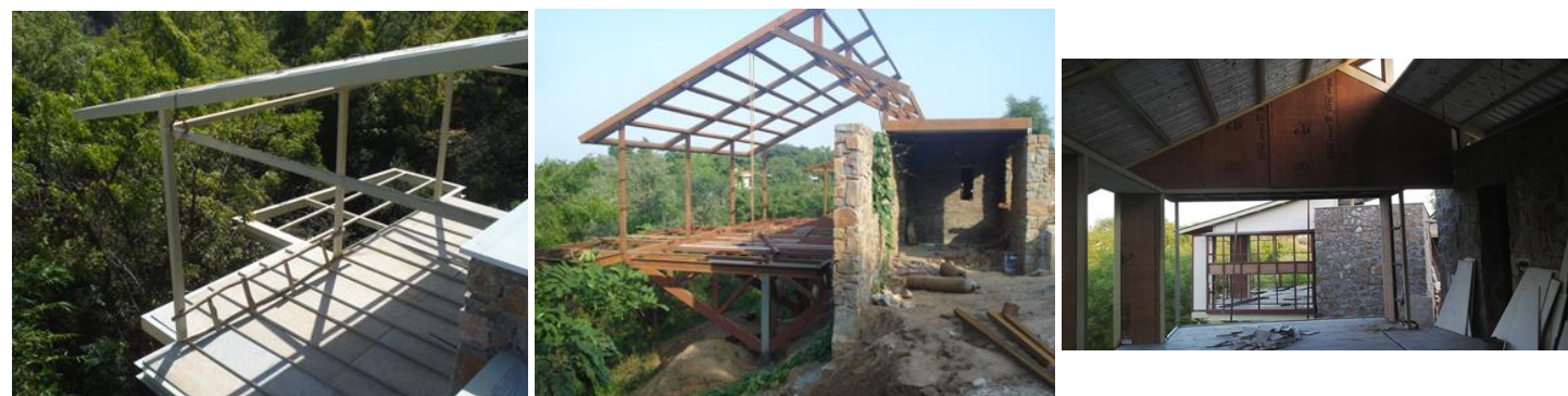
Figure 7 Images of the buildings under construction.
